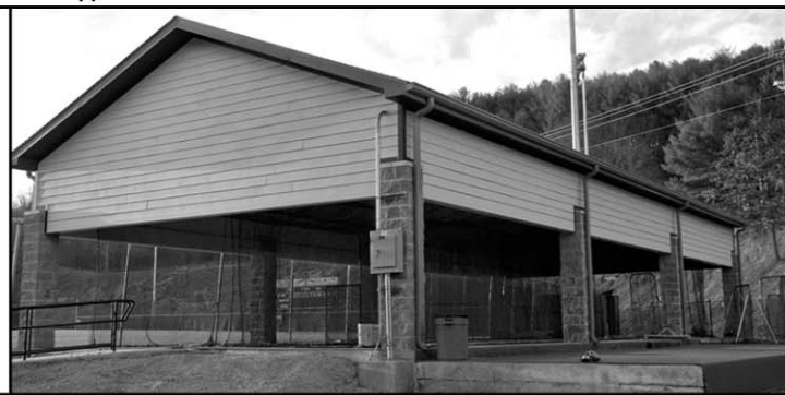
The facility's covered and lighted batting cages lie just beyond the rightfield wall.
